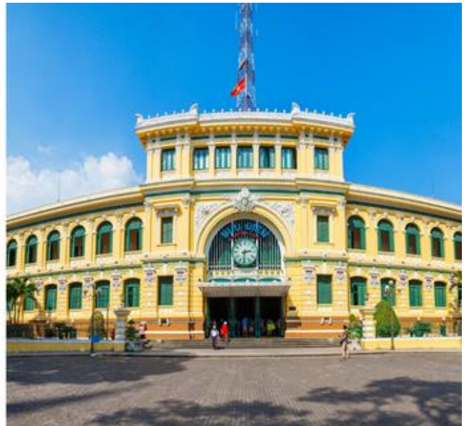
Central Post Office
