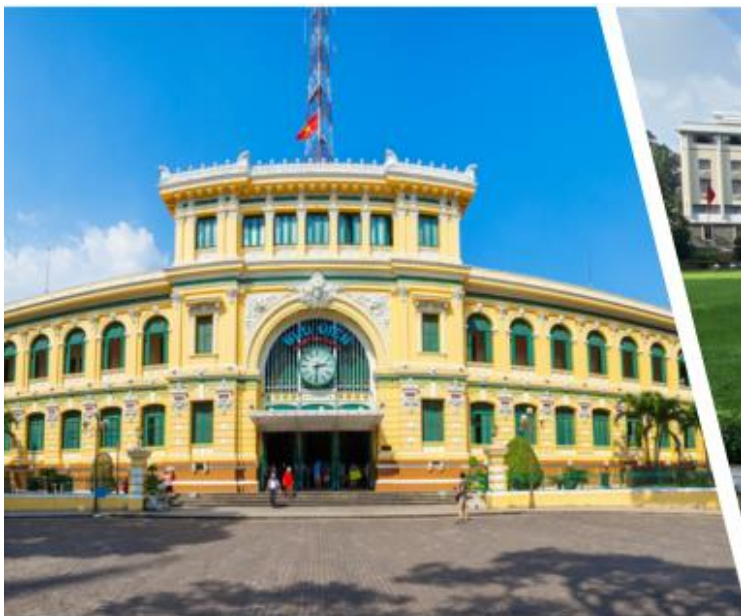
Central Post Office
